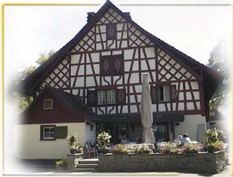
Restaurant Winterthur Eichmühle
